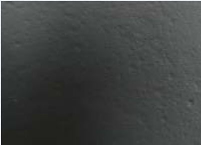
EXPOSE CONCRETE (CECT)
